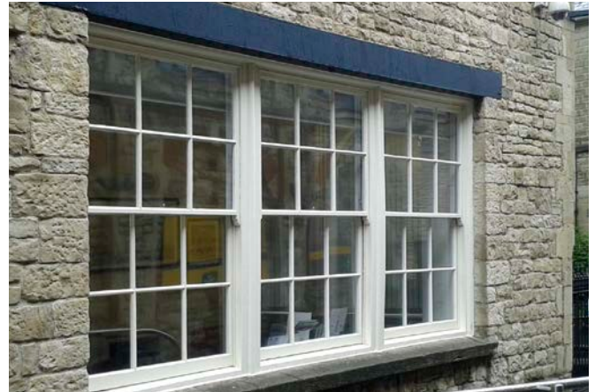
Timber sash windows, The Engine House, Swindon
