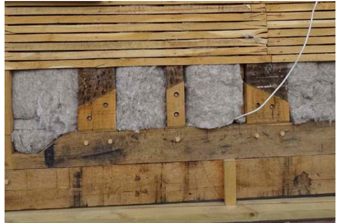
Insulation in timber-framed wall
